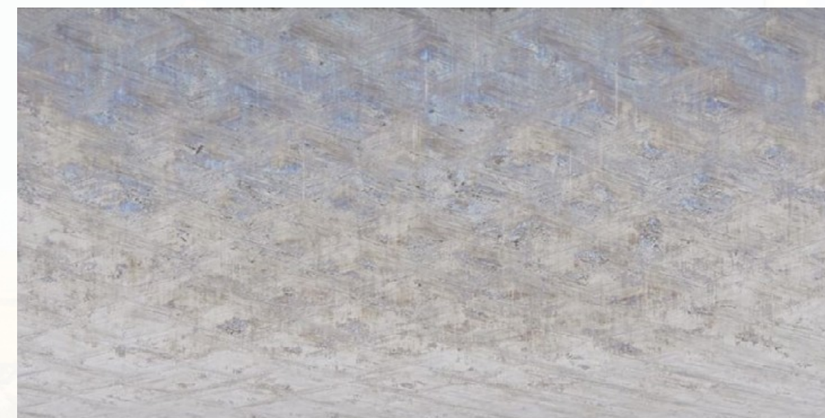
After test completion – like new
